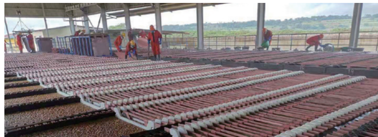
The anode plate equipped with new insulators
