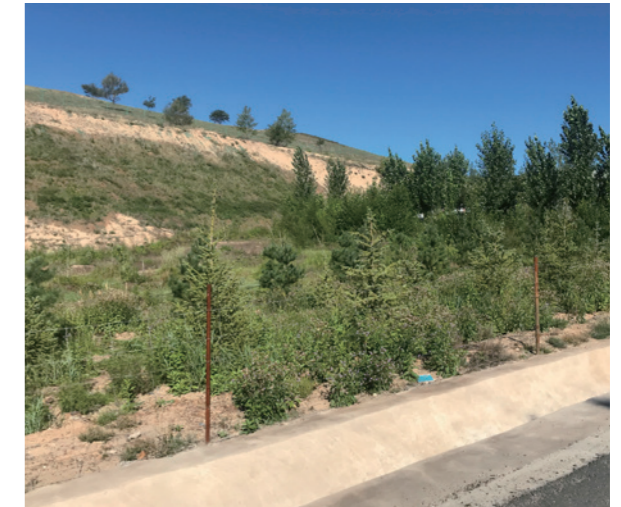
The slope is covered with soil, and planted with grass
