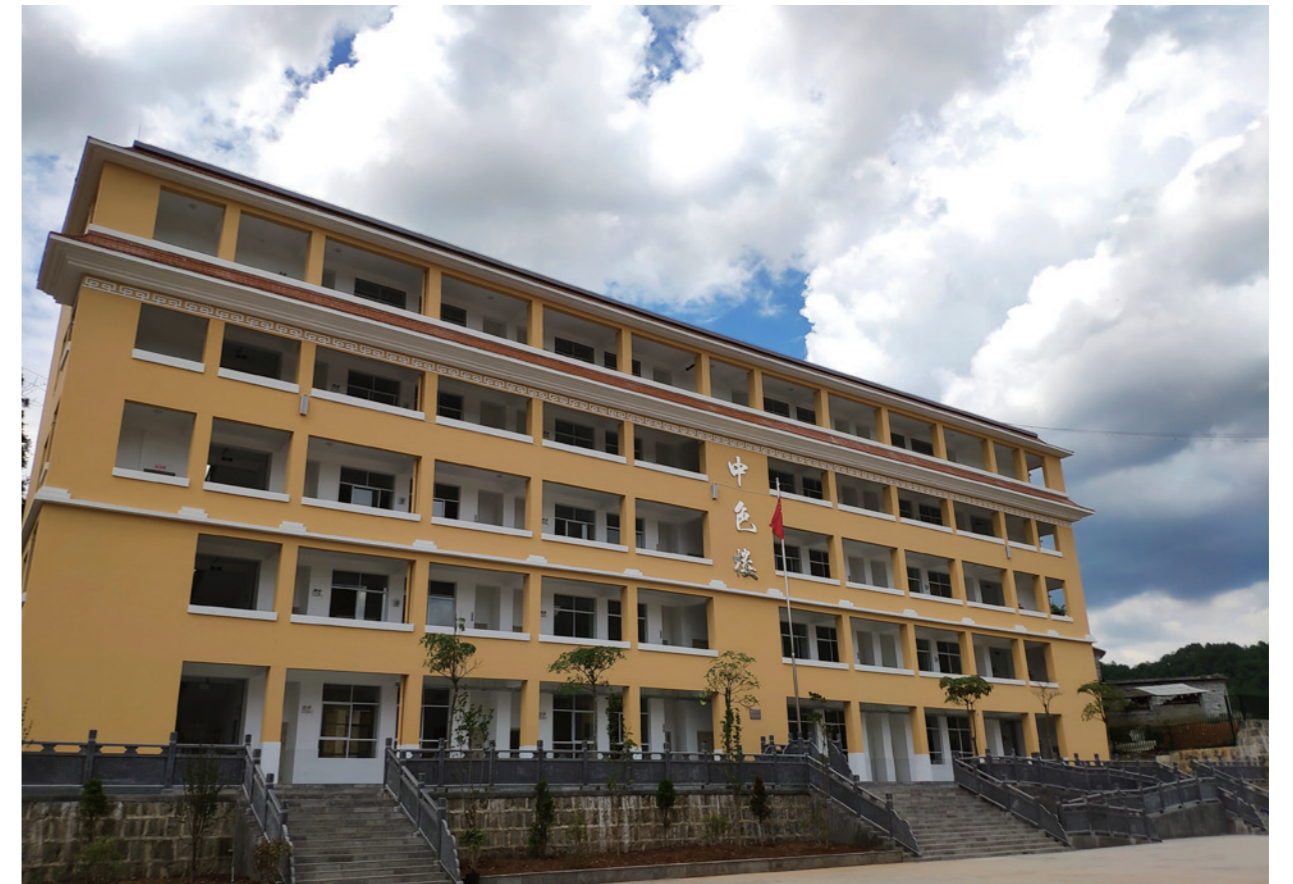
The teaching building of the second elementary school in Mangdong Town, Lianghe County, Yunnan Province, a project for relocation from inhospitable areas built by CNMC
